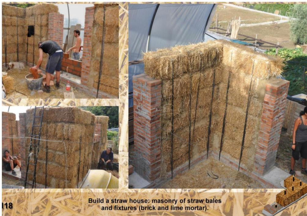
Build a straw house: masonry of straw bales and fixtures (brick and lime mortar).
